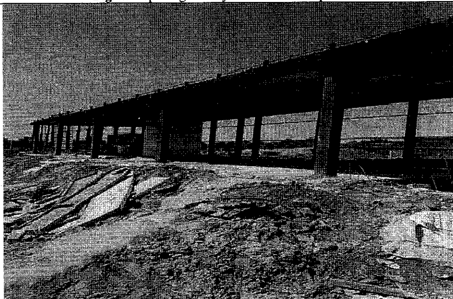
Fig. 2 Depicting civil work for platform for DG sets and water tank.
